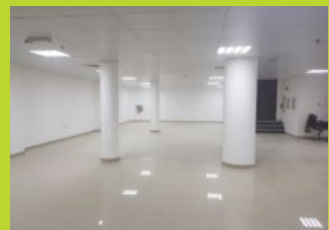
Tiling, Ceiling & Painting
