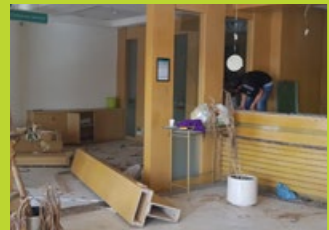
Before & After Demolishing
