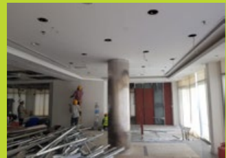
Before & After Demolishing
